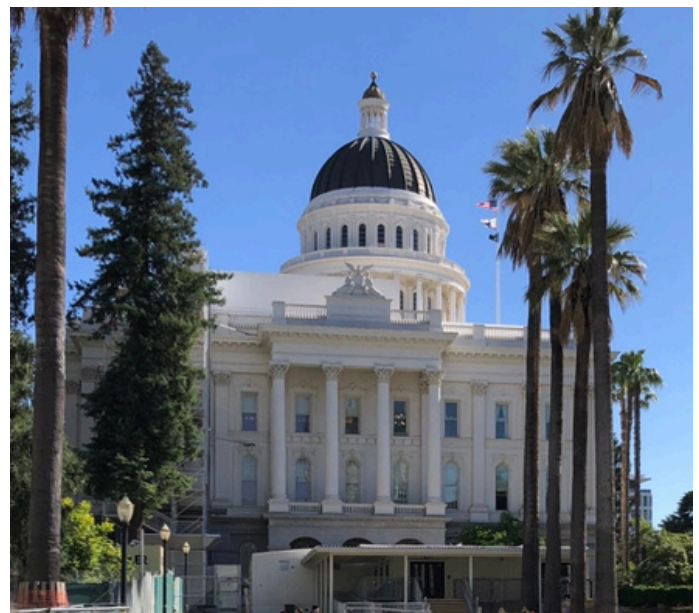
California State Capitol temporary entrance due to Capitol Annex construction.
